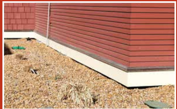
Non-combustible ground cover 5 feet out from combustible structure, the proper treatment of the Home Ignition Zone.
