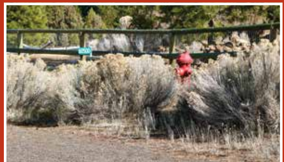
Clear brush 3 feet around all fire hydrants so firefighters can see and access them quickly.
