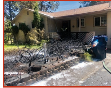
Even a small brush fire can damage a house!
